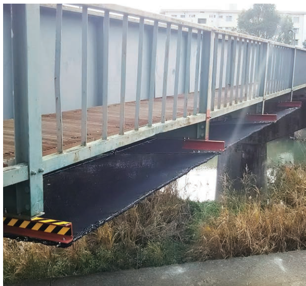
Guard Net for Construction Work
